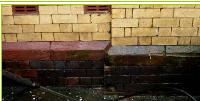
Pink sandstone before (right) and after (left) cleaning reveals its true colour.
